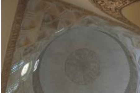
ceiling of mausoleum
